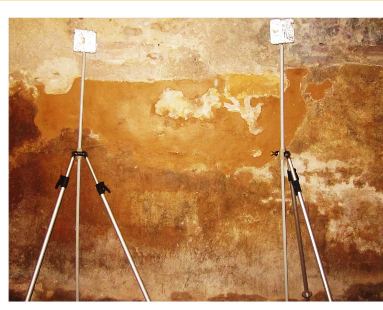
Figure 3: Portion of ancient wall analyzed by thermographic data acquisition. Yellow-brown area is a past unknown restoration.
