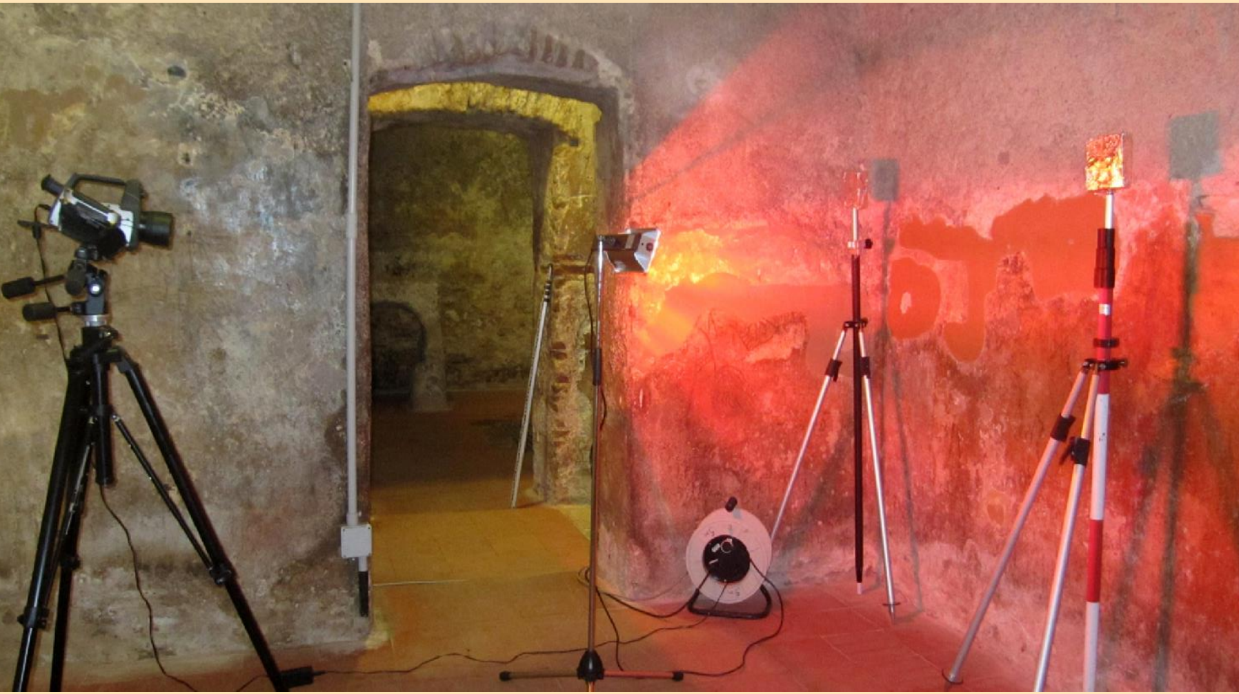
Figure 2: Thermographic data acquisition. Thermographic camera-on the left; electrical infrared heater-in the middle; reflecting targets-on the right.
