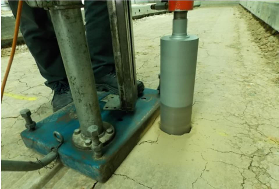
**FIG. 9** – Extraction of drill cores.
