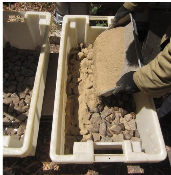
**FIG. 6 – Distribution of soil between two consecutive layers of ballast.**
