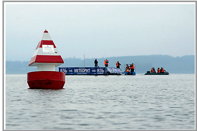
Fig. 17. Floating platform for diving works.
